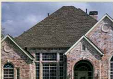
The same roof again, on an overcast day.
