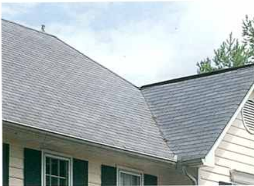
Ordinary three-tab shingles are so flat and thin they allow roof deck imperfections to show through.
