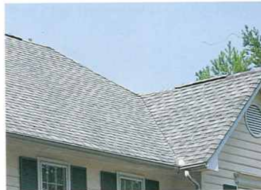
Elk Prestique Plus 40 High Definition shingles mask roof deck imperfections and give the same home a more distinctive look.
