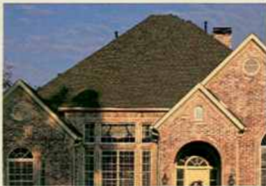
The same roof in full sun during the late afternoon.
