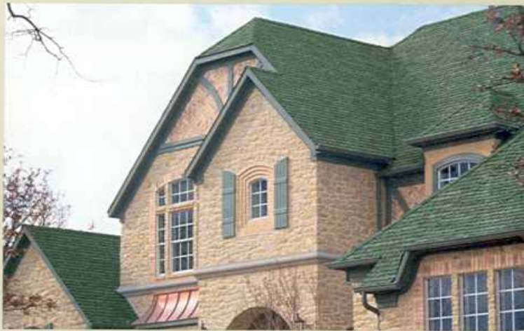
Capstone 40 in new Village Green.
